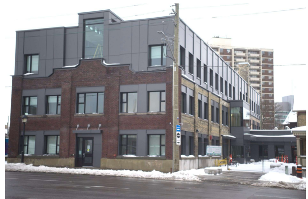
Top: Port Hope. Commercial building with upper floors converted to residential use. Bottom: Kitchener. Former button factory converted to supportive housing units.
