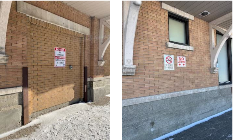
Face brick detailing, openings, concrete foundation and eave brackets. Photos: N Alexander, April 2023
