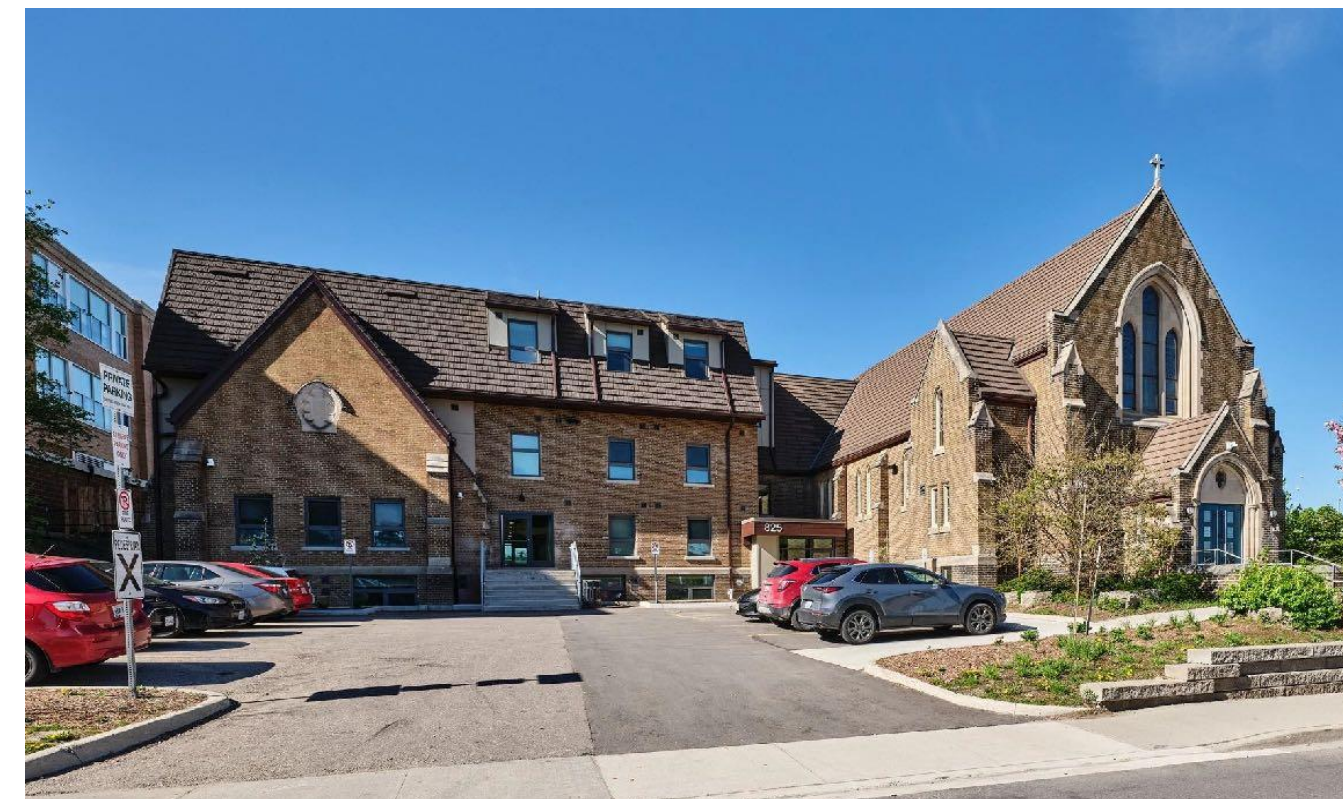
Church to supportive housing at St. Mark's Place in Kitchener: Recipient of the ACO Paul Oberman Award for Adaptive Reuse, 2024
