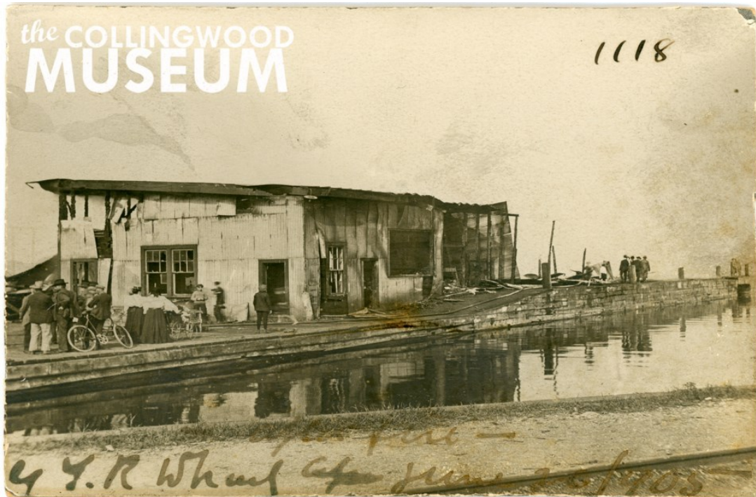
Figure 22 – Damage to the freight sheds from the 1905 fire (Source: Collingwood Museum, n.d. b)
