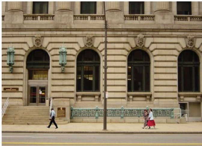
PERSPECTIVE VIEW AT SUPERIOR AVENUE, MAIN BUILDING ENTRANCE BEFORE
