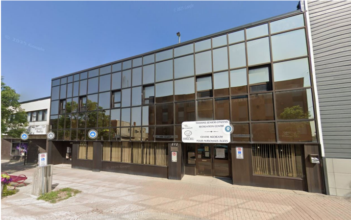
The H.R. Bielek building located at 272 Third Avenue, which presently houses the Timmins Senior Citizens Recreation Centre. The original façade of the New Empire Theatre is obscured behind a metal and glass curtain wall that was installed in the 1980s (Google Street View, August 2024).
