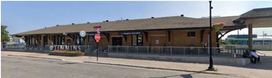
West Elevation – Google Street View (August 2024)
