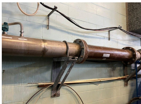
The influent piping that contains the static mixer
