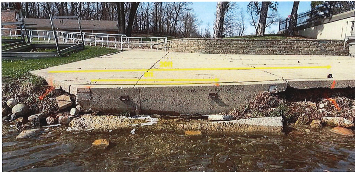
Current view – 8ft pier / 20- 30ft of rip rap area; Proposed Rip Rap Below
