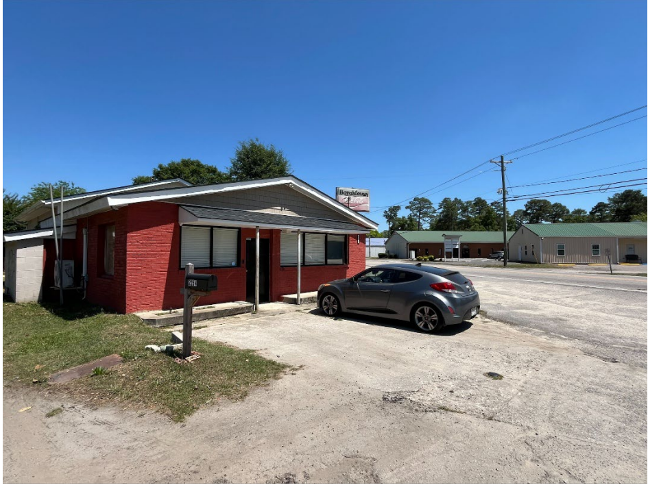
Existing structure on subject parcel.
