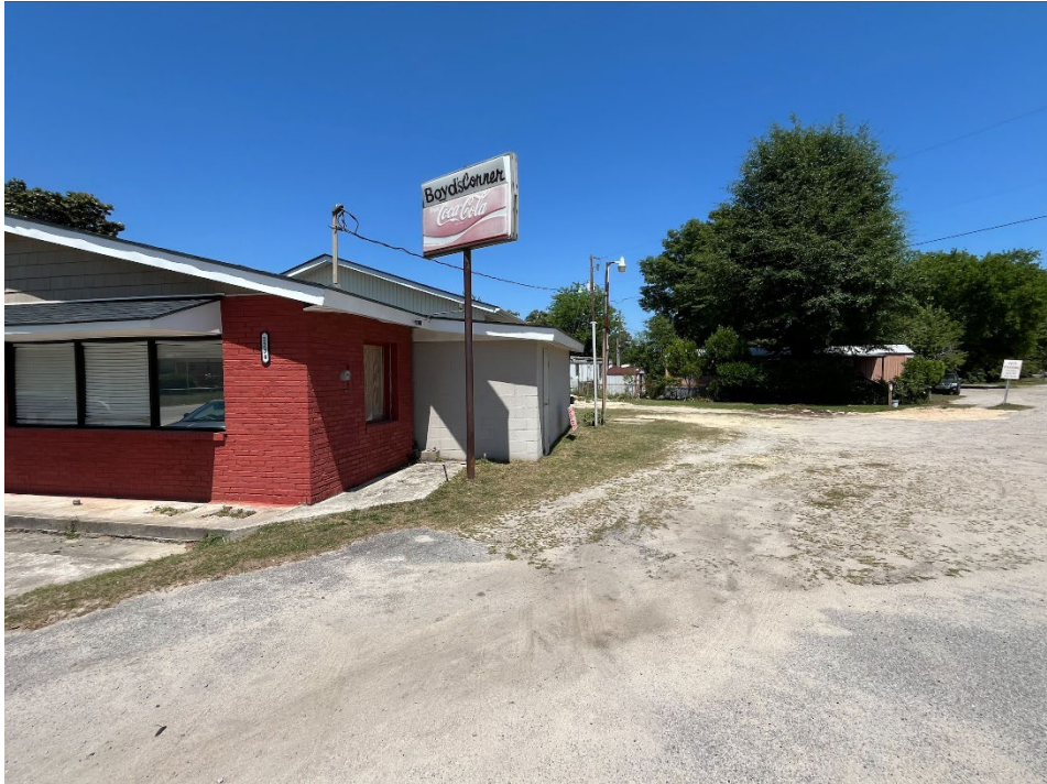
Existing structure on subject parcel.
